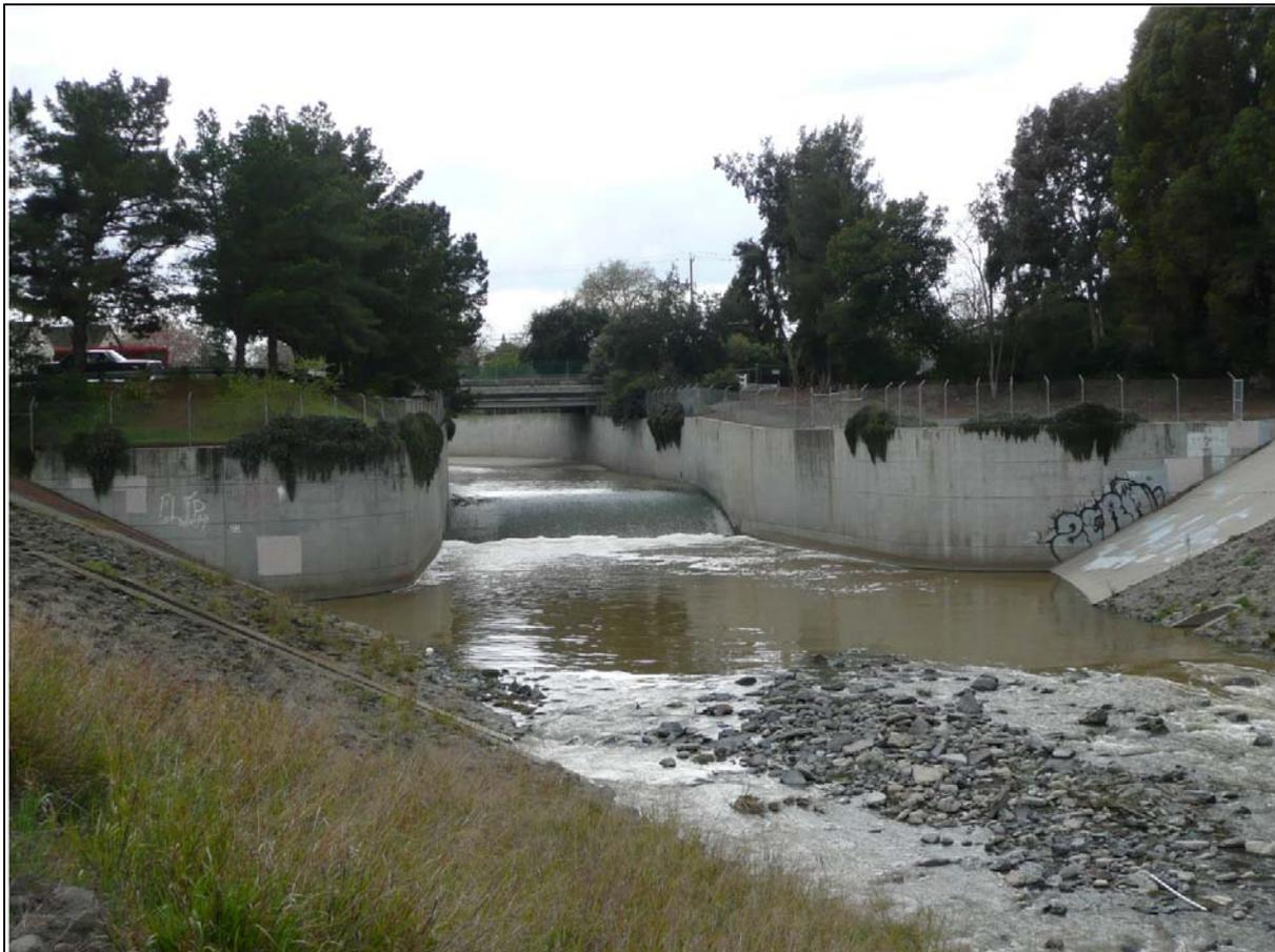
Figure ES-1. Drop Structure 2 at a Relatively Low Flow
