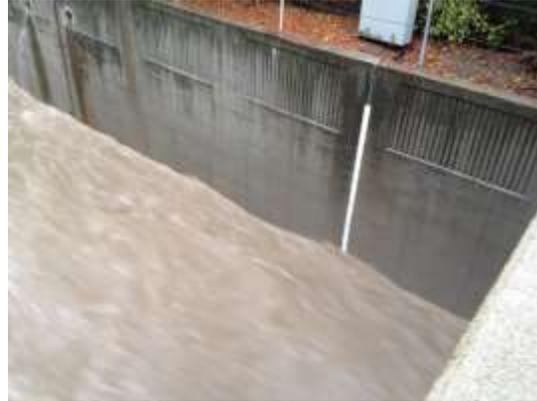
The FC District also installed a stream gauge on Marsh Creek near the Sheriff's Detention Facility off of Marsh Creek Road in January 2010. We have not established a rating curve for this gauge either.
