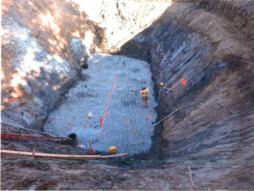
Abutment 2 footing excavation with drain rock placed.
