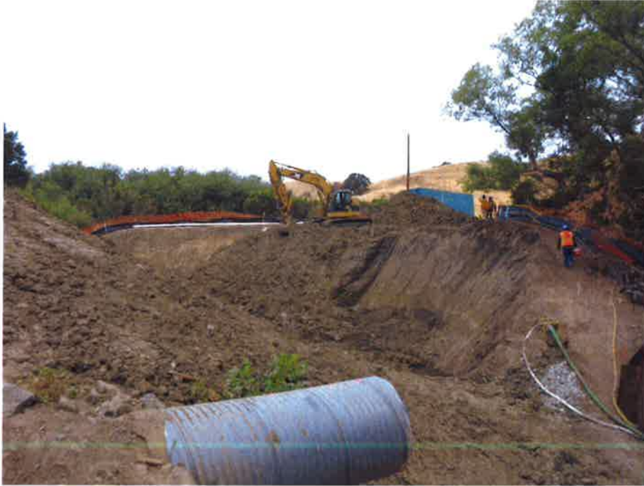
Abutment 2 footing excavation continues.
