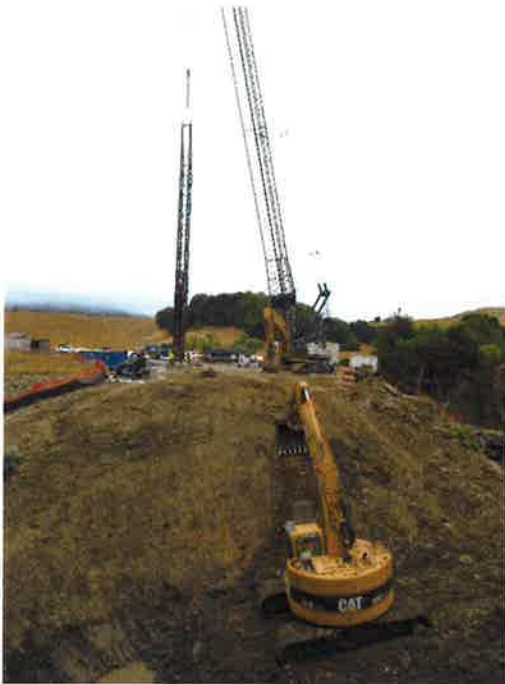
Excavation for Abutment 2 and crane pad.
