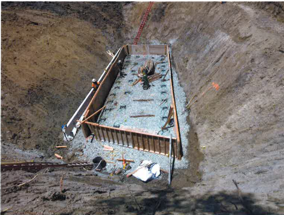
Footing forms being installed at Abutment 2.
