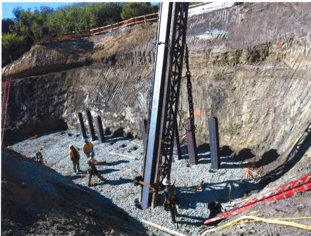
Batter piles being driven at Abutment 2 footing.
