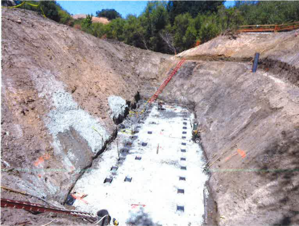
Pile driving operation complete at Abutment 2 footing.
