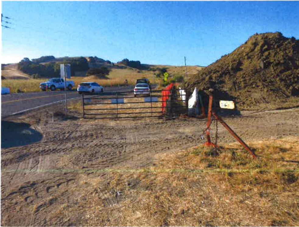
Soil stockpile at EBMUD property.
