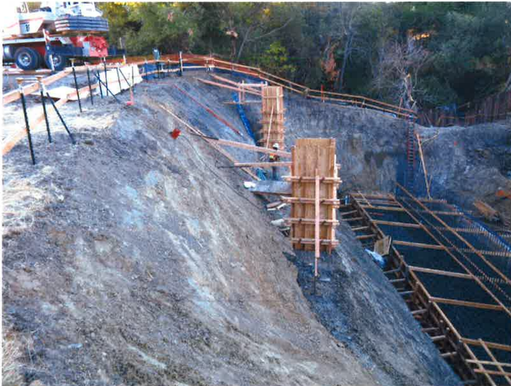
Abut. 2 wingwall piles concrete extension form work.
