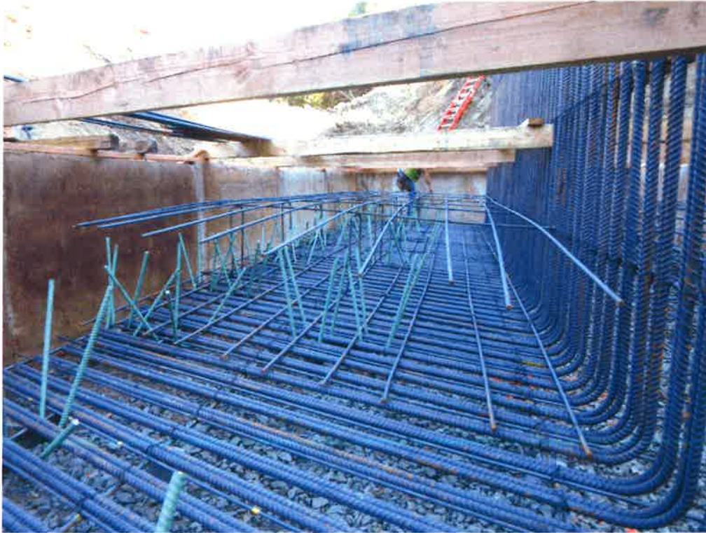
Rebar being installed Abut. 2 footing.
