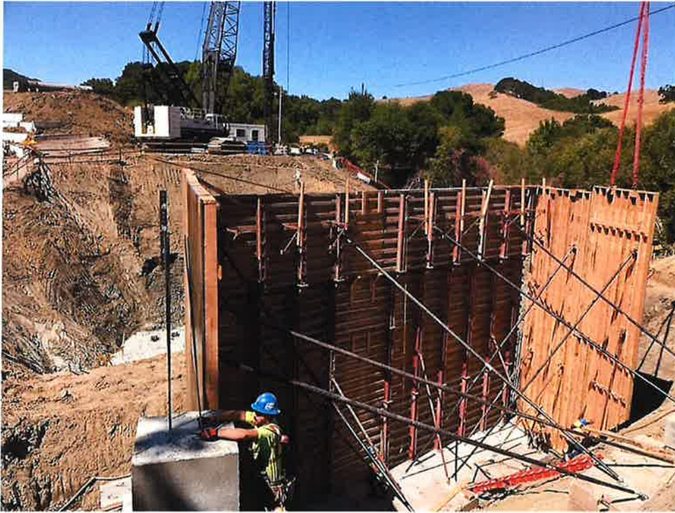
Abut. 2 stem forms being installed.
