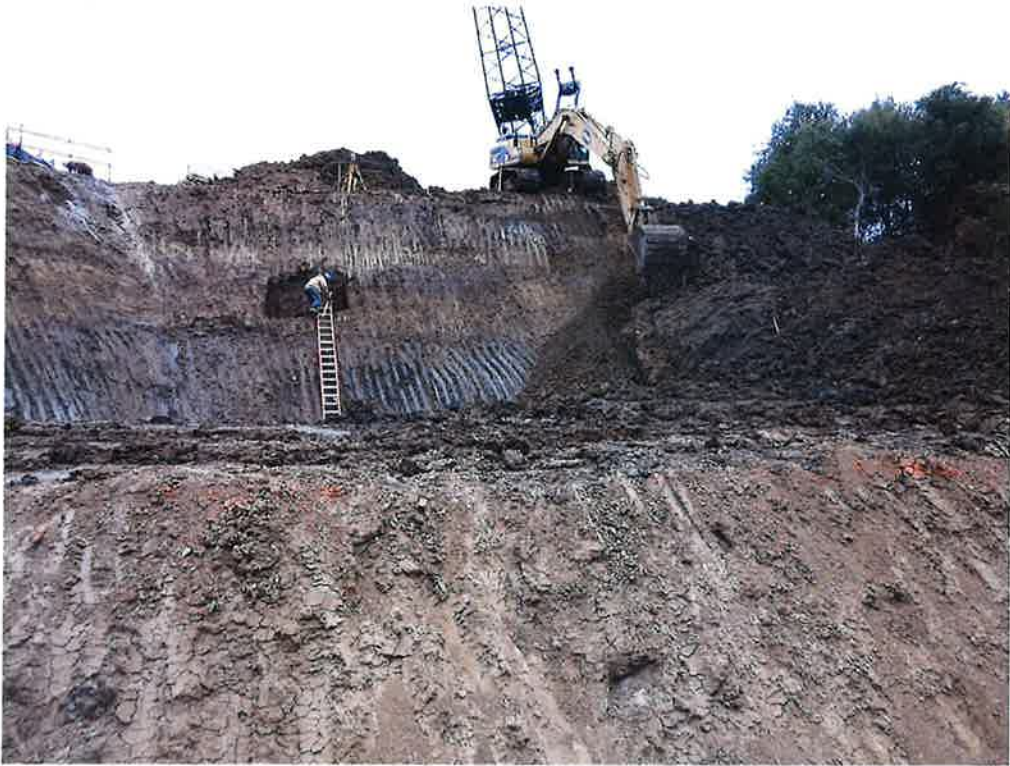
Abut. 1 excavation continues.
