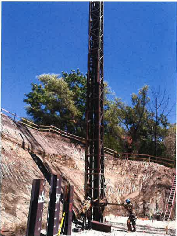
Abut. 1 pile driving.
