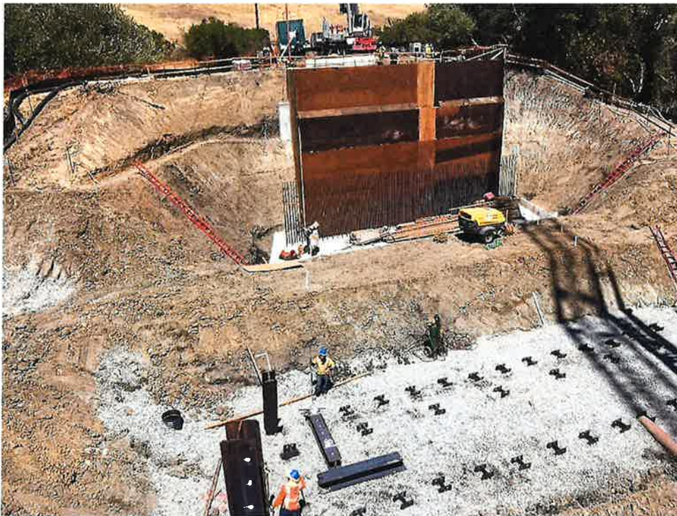
Abut. 1 piles and Abut. 2 formwork.
