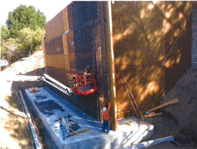
Abut. 2 reinforcing bar being installed.
