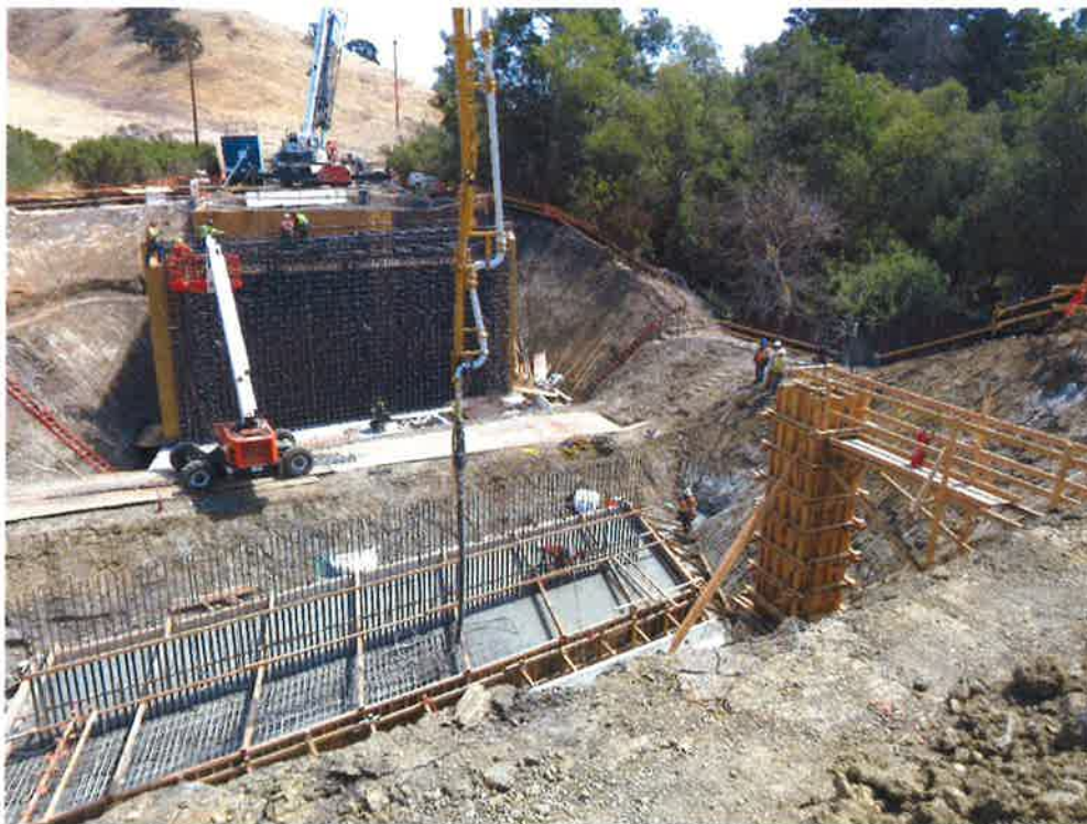
Abut. 1 footing pour and Abut. 2 reinforcing bar being installed.
