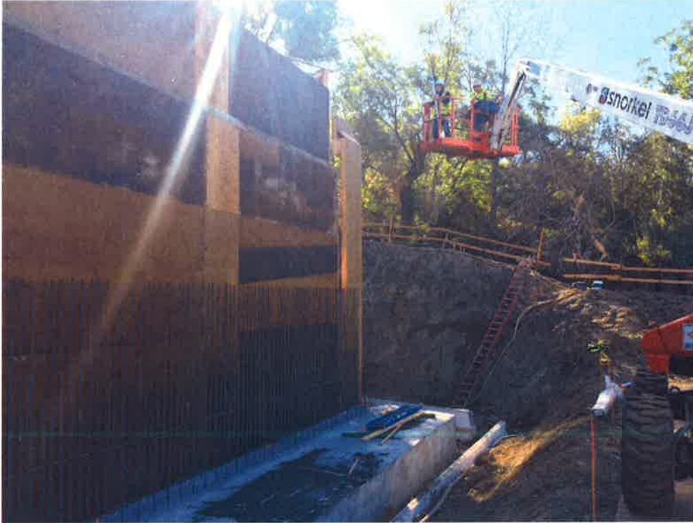
Abut. 2 seat and wingwall grade check.
