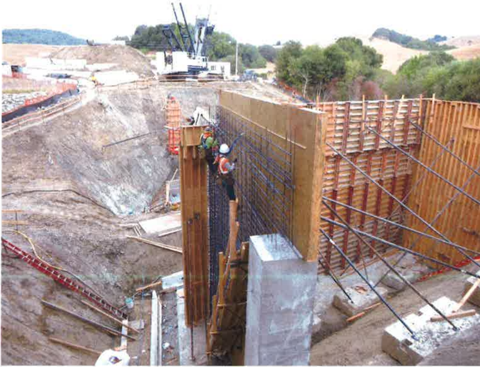
Abut. 2 wingwall reinforcing bar being installed.
