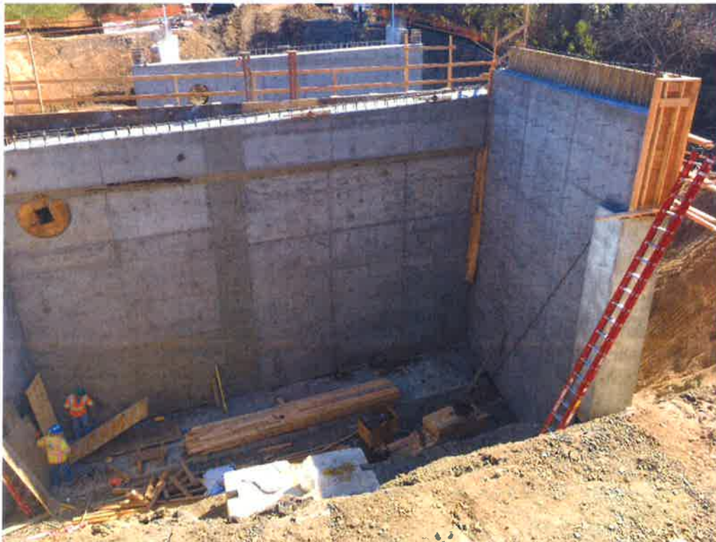
Abutment 1 stem (back of Abutment) stripping.
