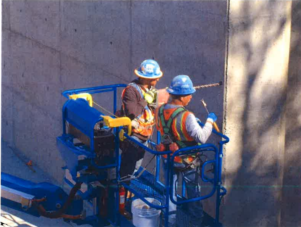
Abutment 2 face being patched.
