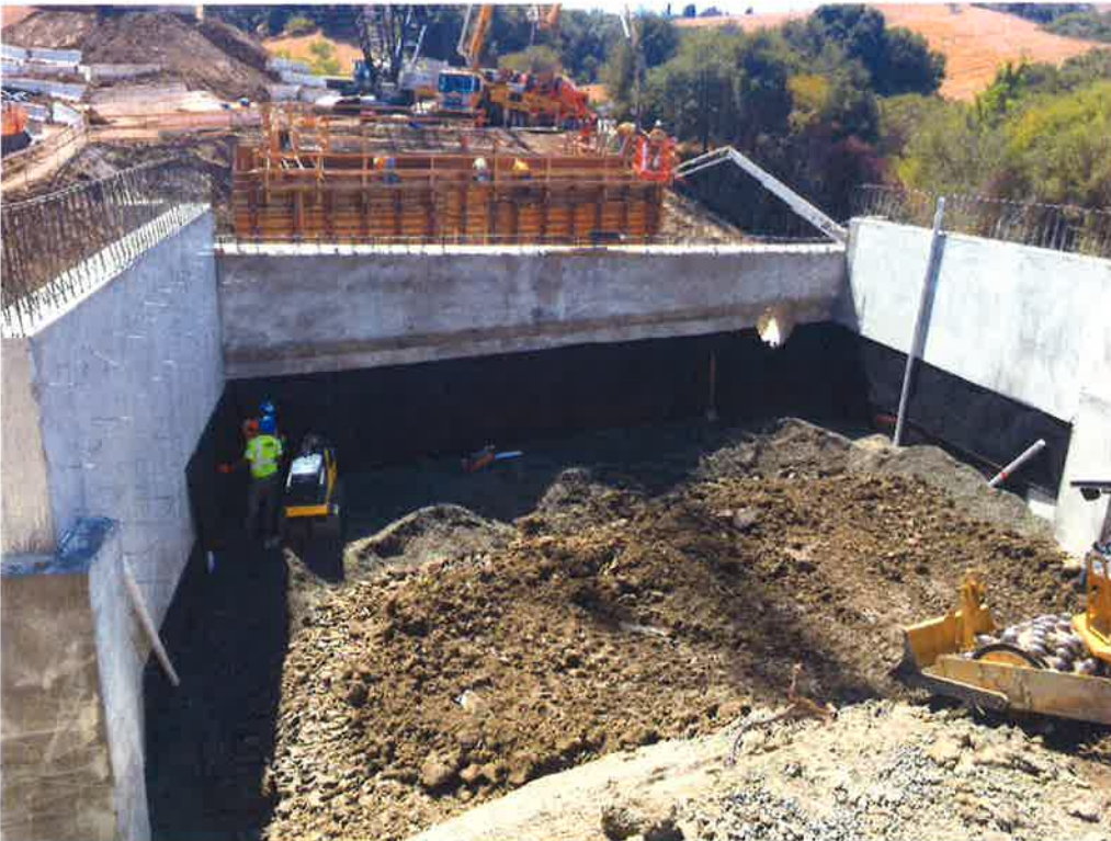
Abutment 2 backfill and hydro duct being installed.
