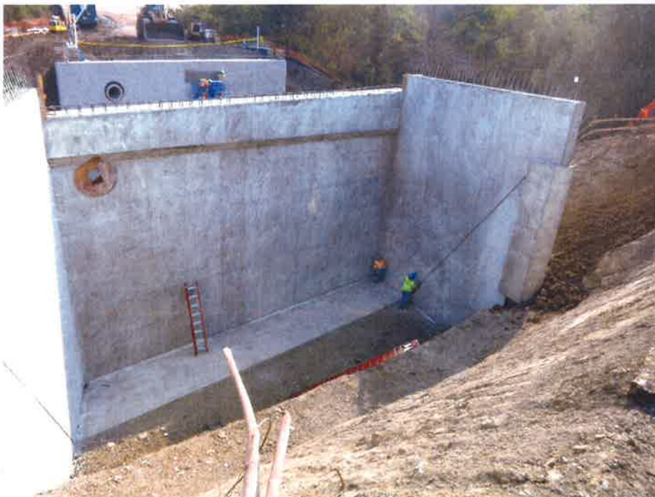
Abutment 1 patching the back face, and abutment 2 patching in the background.
