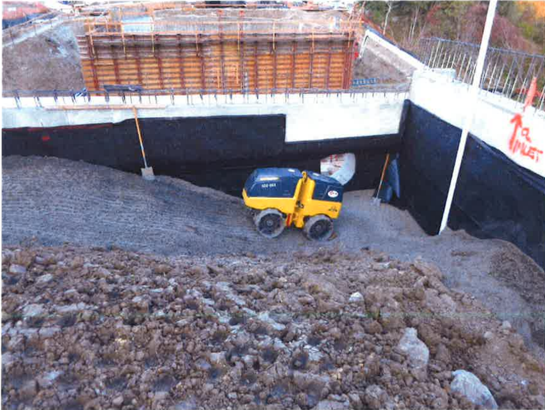
Abutment 2 structure backfill.
