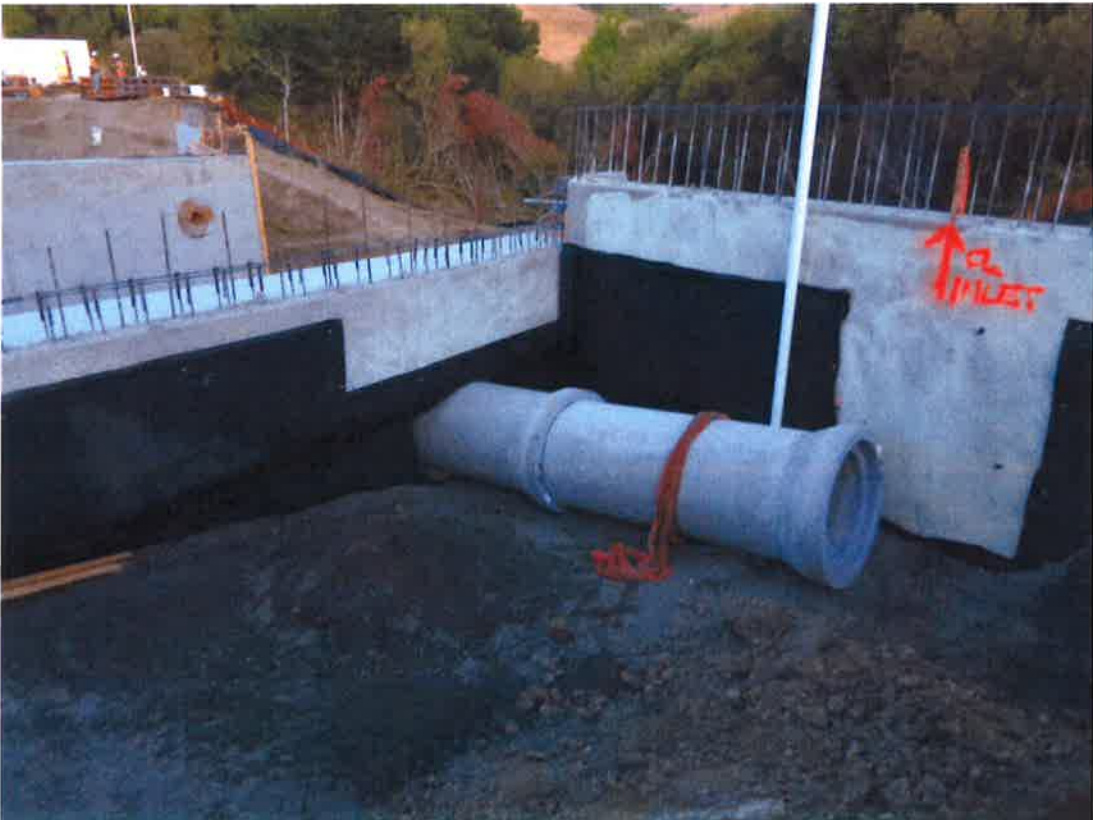
Abutment 2 drainage system being installed.
