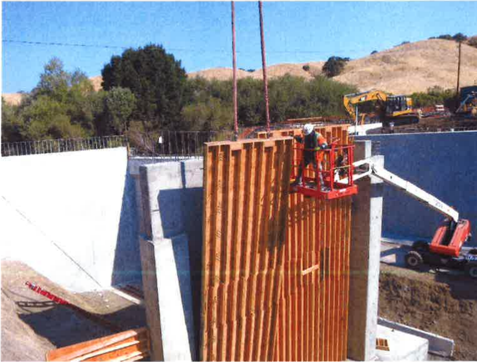
Abutment 1 stripping the wingwalls.
