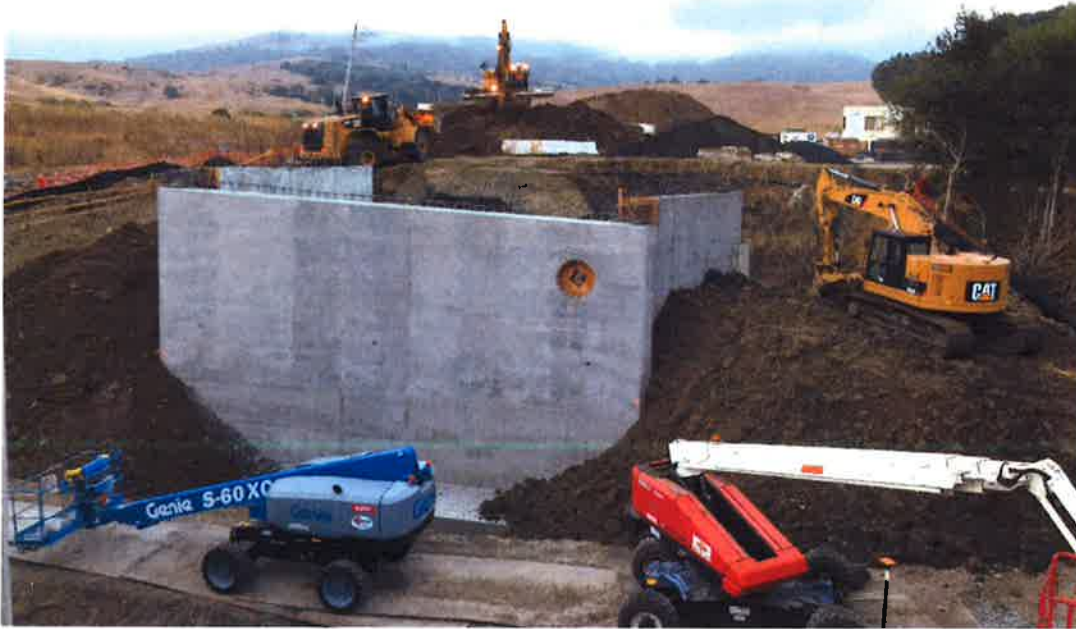
Soil being moved from stockpile to various locations throughout project.
