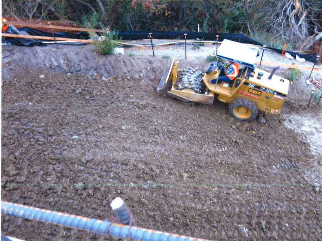
Backfill at abutment 2 outside of the wing walls.
