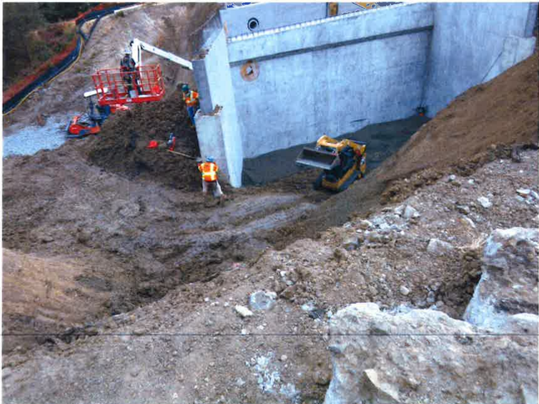
Abutment 1 structure backfill and class 1 surface finishing of the wing walls.
