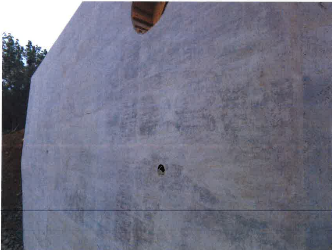
Abutment 1 stem (Class 1 surface finish).
