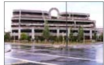
Masking the large parking garages will be critical to making this an active, pedestrian-oriented town center.
