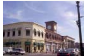
Parking garages in downtown Walnut Creek are articulated with upper story windows that relate to the older buildings in town.
