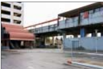
The existing taxi area.
